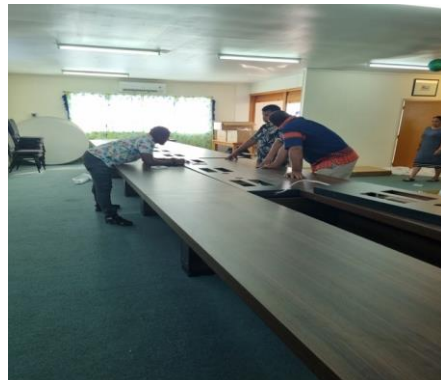
Technicians and Nauru Parliament ICT staff discussing the installation of the video conferencing equipment
